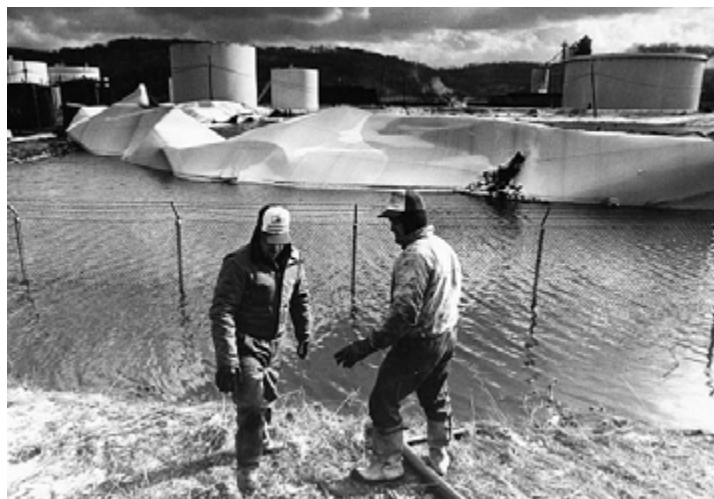
Figure 33: Cleanup Workers at Ashland Storage Yard in Aftermath of Tank Collapse 92
