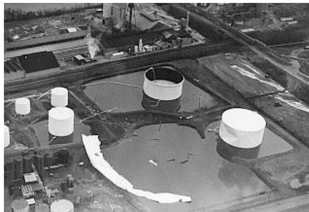
Figure 32: Aerial Photo of Collapsed Ashland Oil Tank
