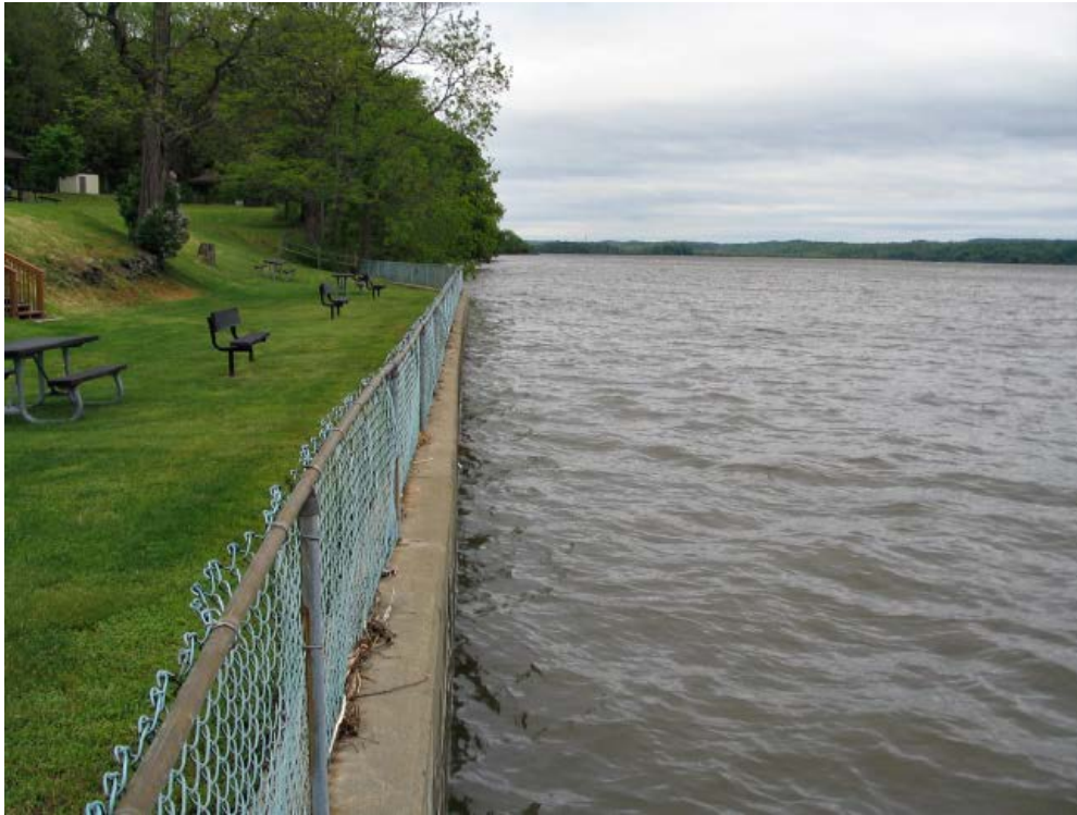
Figure 44: ESI 8B S Sheltered Man-Made Structures on Hudson River
